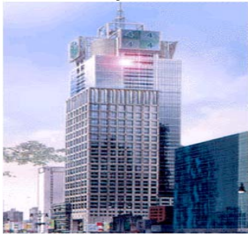
Four Times Square: The first building built in New York in the 1990s using modern energy efficiency guidelines.
