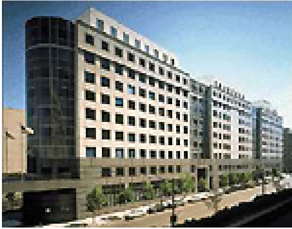
The Aerospace Center, an Energy Star® Building, at Washington D.C.'s L'Enfant Plaza.
