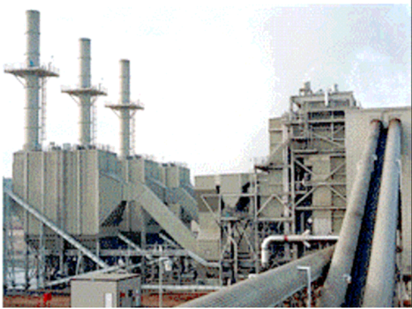
Biomass electric plant in Anderson, California.
