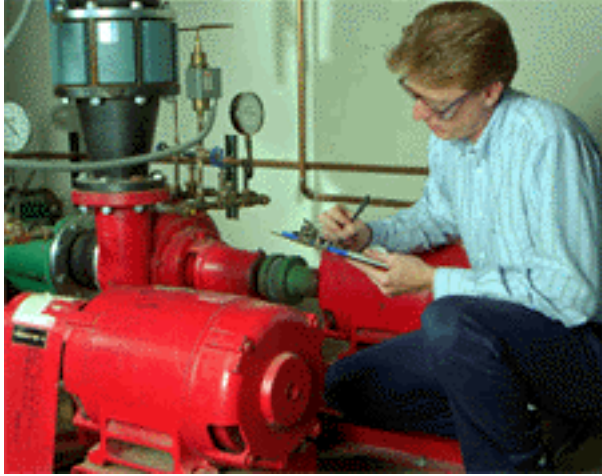
Replacing an inefficient motor.
