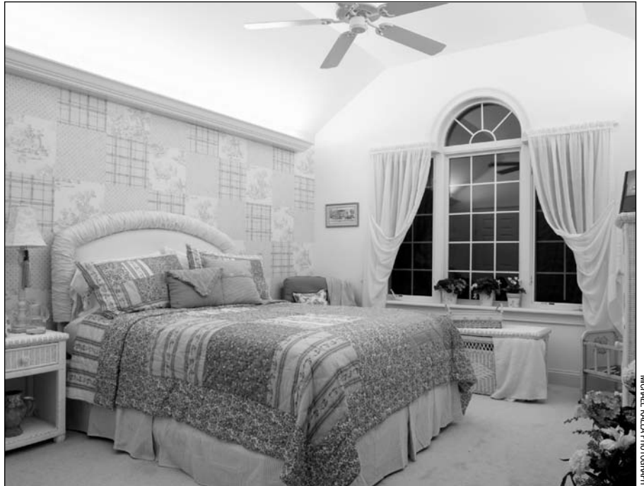
Custom-built cove lighting directs light upward, enhancing the appearance of vaulted ceiling and providing glare-free general lighting.
