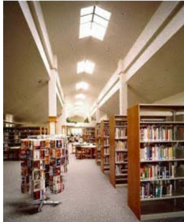
Linear skylight in this library spreads daylight to adjacent spaces and organizes the circulation
