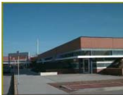
Photo of Liberty Elementary School with exterior lightshelves to reflect sunlight onto classroom ceilings. Photo courtesy of Liberty Elementary, Boise School District, Boise, ID
