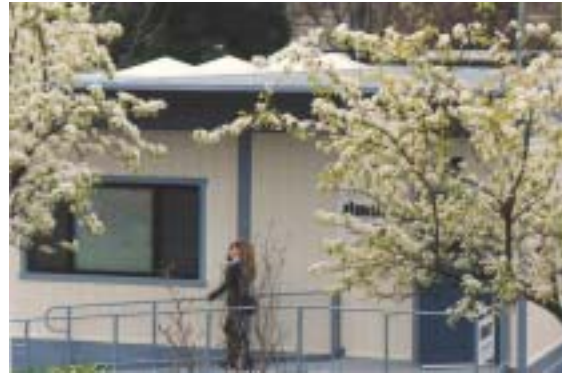
Pyramid skylights on experimental portable classroom design integrates skylights into a high efficiency modular design. Photo courtesy Lisa Heschang.
