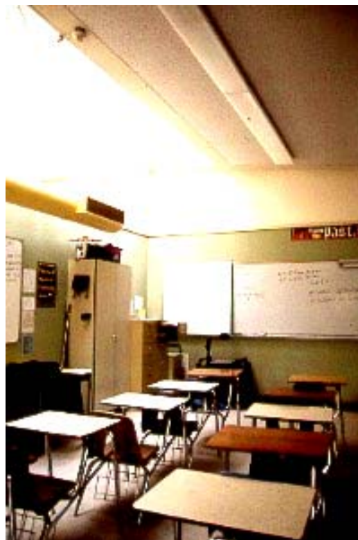
Skylit wall wash delivers daylight across two-thirds of this classroom. Lisa Heschong, photographer.
