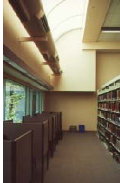
View windows at RI library are separated from the daylight feature overhead and use lower transmission glass to reduce glare. Lisa Heschong, photographer.
