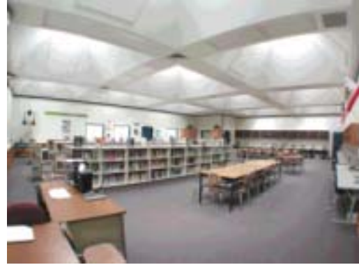
Deeply coffered ceiling helps to diffuse light from four skylights. There are no electric lights on in this photo. Photo courtesy SunOptics.
