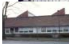
Central sawtooth monitor provides even illumination across desktops in this classroom. Photo courtesy: Barbara Erwine.
