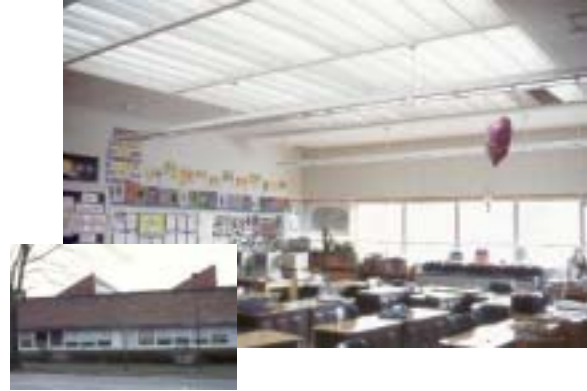
Guideline DL5: Central Toplighting from a sawtooth monitor with sun baffles is combined with DL1: View Windows to provide balanced illumination in a classroom. Photos courtesy Barbara Erwine.
