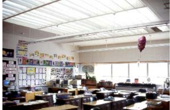
Gentle, diffuse daylight permeates a classroom with both sidelight and toplight. Note that all surfaces are painted white to distribute light more efficiently and reduce contrast glare. Photo courtesy Barbara Erwine.
