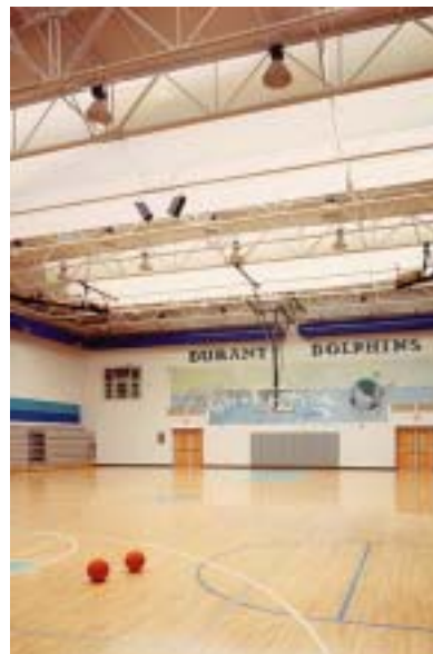
Monitors provide diffuse light into gymnasium at the Durant Middle School gym. Photo courtesy Innovative Design.
