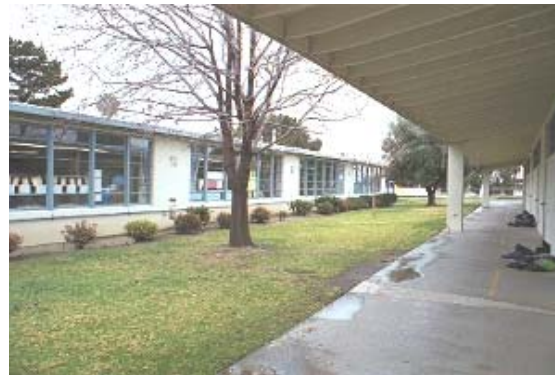
North versus south windows. South windows are shaded from direct sun, but receive daylight reflected off of concrete walk and white painted overhangs. North windows are large and unshaded. Photo courtesy Lisa Heschang.
