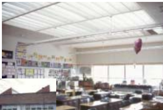
Central sawtooth monitor provides even illumination across desktops in this classroom. Photo courtesy: Barbara Erwine.
