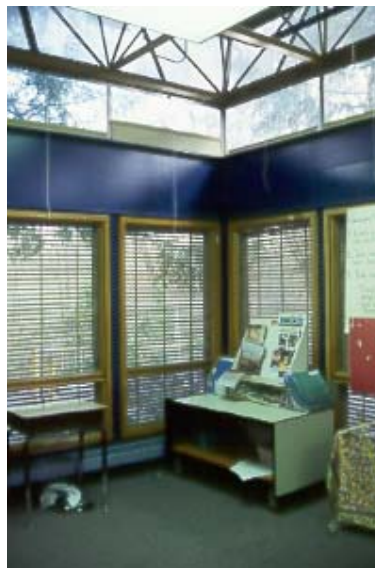
Horizontal blinds allow control of brightness from lower view windows. Note that high clerestory windows have no blinds so that daylight can reach deep into classroom. Most classrooms do not need complete black out capability for viewing of modern video equipment. Photo courtesy Barbara Erwine.
