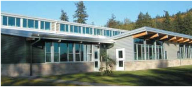
The Riverview Elementary School, Lebanon, OR, puts light where people need it the most through perimeter daylighting and skylights.
