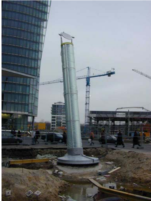
Figure 6: One of the lightpipes at Potsdamer Platz during installation [Signer, 2002].
