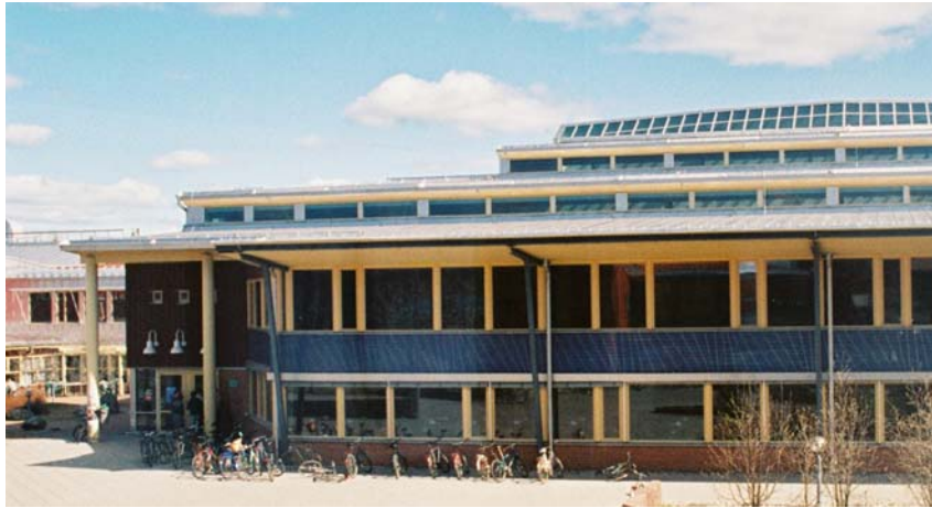
Figure 9: Toplighting at the library building of Luleå University of Technology. There are two rows of clerestories below a 45° monitor furthest away on the sloped roof. The light from the monitor falls onto the back wall of the library, which acts as a diffuse reflector.
