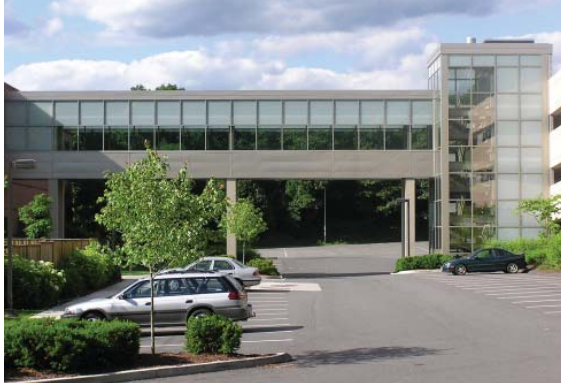
It is quite common to specify luminaires with different distribution in the same parking area. The luminaires can still have the same outward appearance and use the same lamp.
