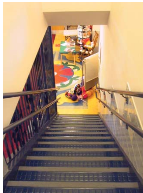
Lighter-colored band on nosing makes steps more visible.
