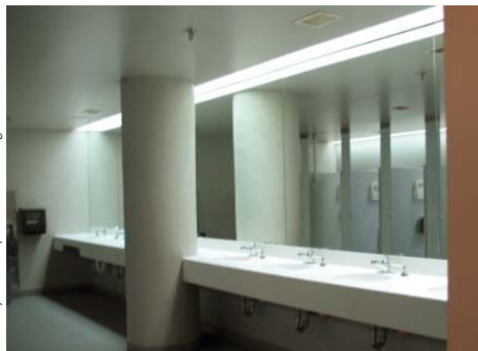
Lighting is primarily needed at the perimeter walls of restrooms -- over mirrors, sinks and toilets.
