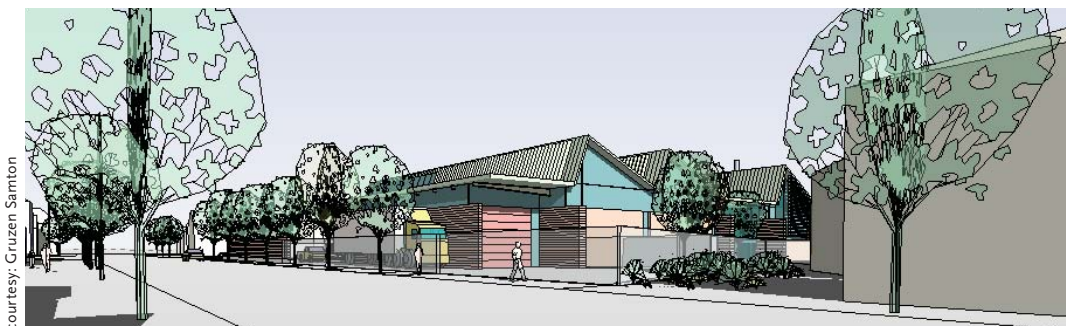
North-facing monitors and angled louvers ensure that daylighting is the primary source of light for the workshops at Sunrise Yard. The direct sunlight is never allowed to hit the work surfaces during work hours.
