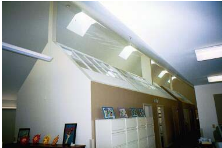
Figure 2. Quabbin Project – Interior Roof System
