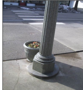
Concrete Pole (Over 20 Years Old)
