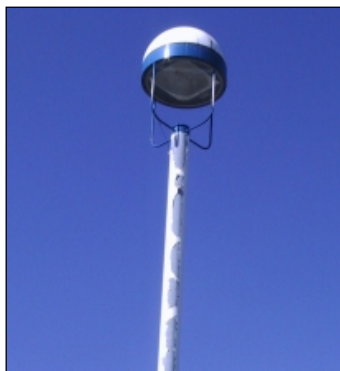
Poor Powder Coating
