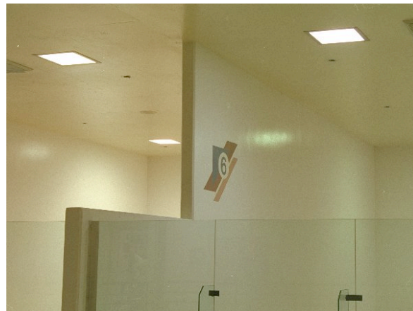
Photos of a racquetball court. Note how much brighter the court is after the T5HO system retrofit (shown on the left side).
