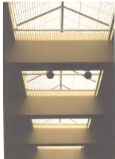
*Linear skylight in multipurpose room includes electrically operated louvers to reduce brightness when needed. Photo courtesy Lisa Heschong.*
